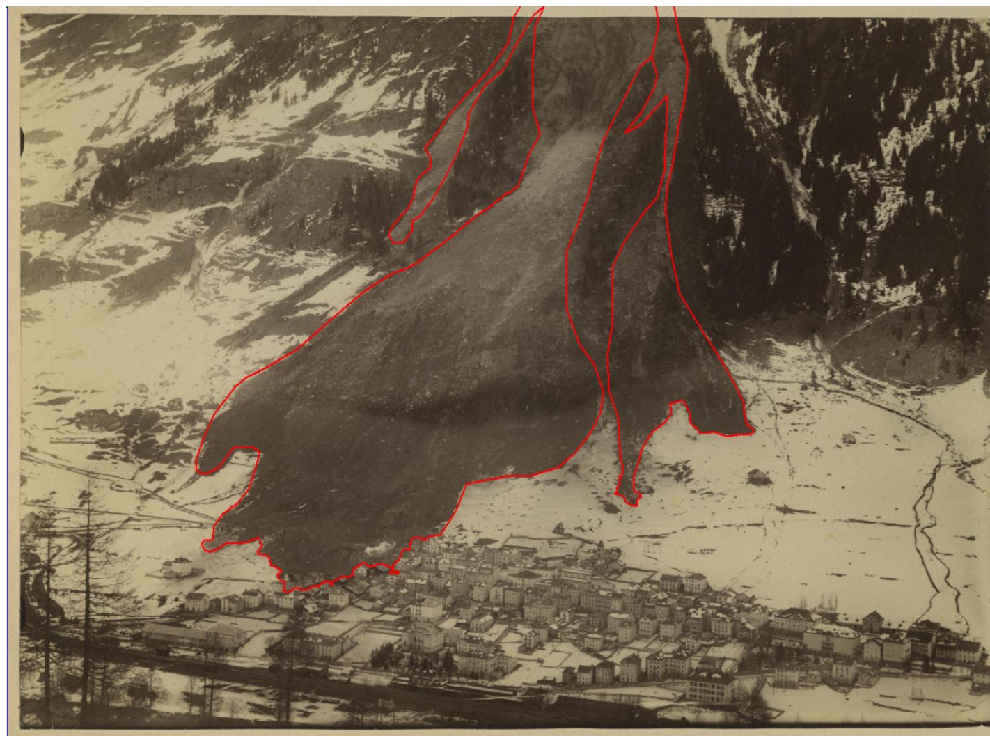
Partial photograph on the rockslide area.
